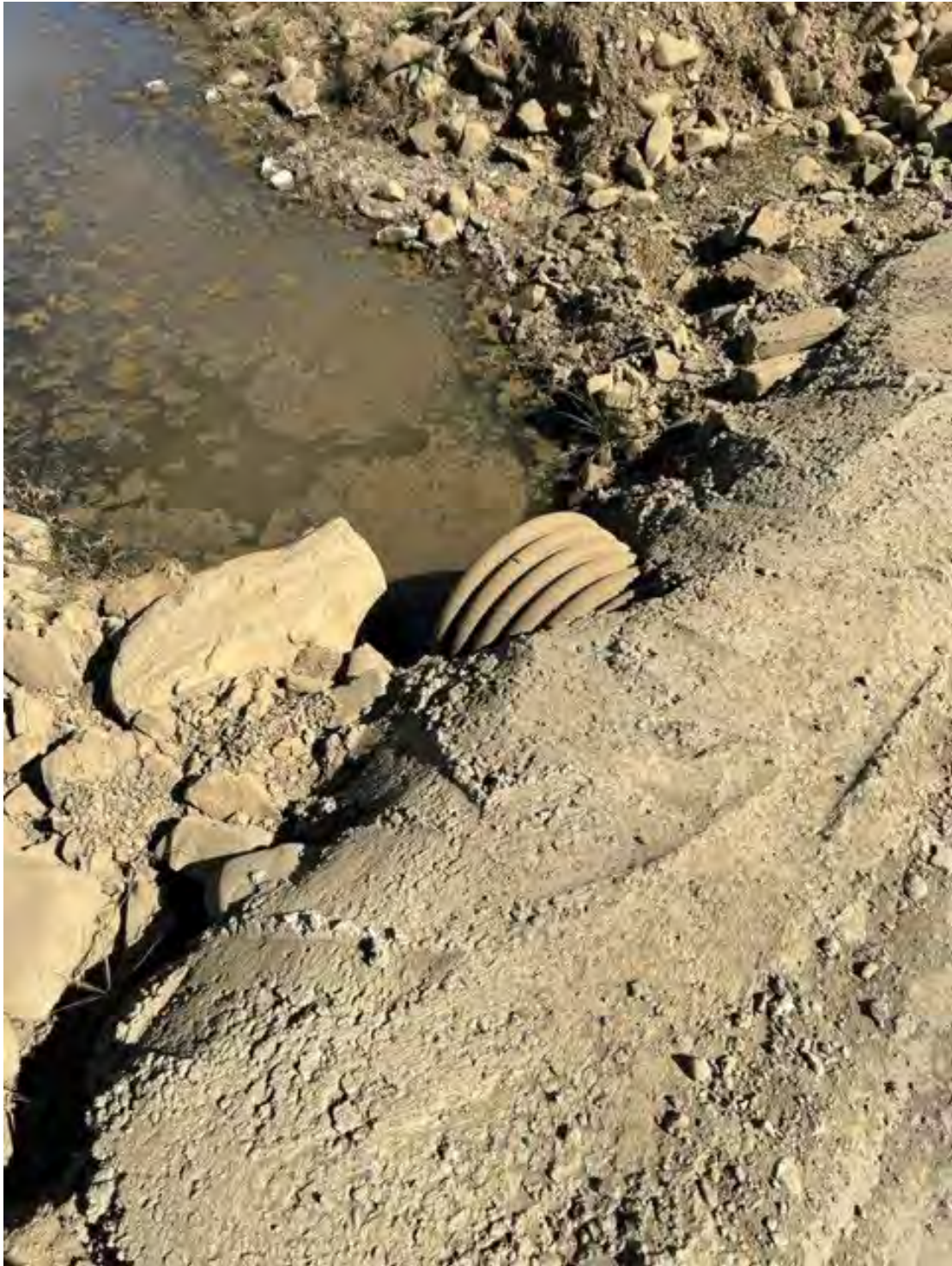
Plate 12: Pipe Culvert in the Creek Crossing on Rannock Burn Road.
